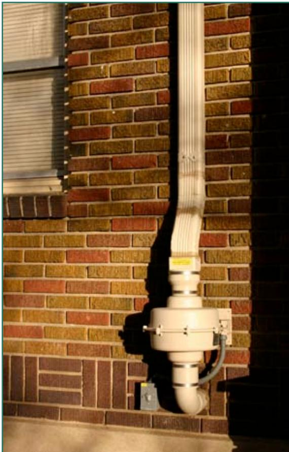
*Radon vent system installed on an older home. It is a sub-slab suction system that reduced the basement radon level from 6.4 pCi/L to 2.6 pCi/L.*
