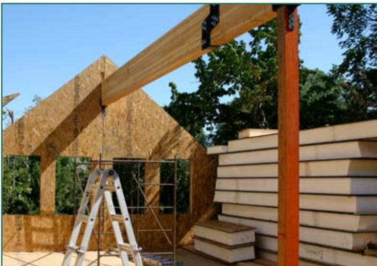
Picture above shows a SIP wall, glu-lam ridge beam, LVL column and 10-inch thick SIP roof panels on far right side of photograph
