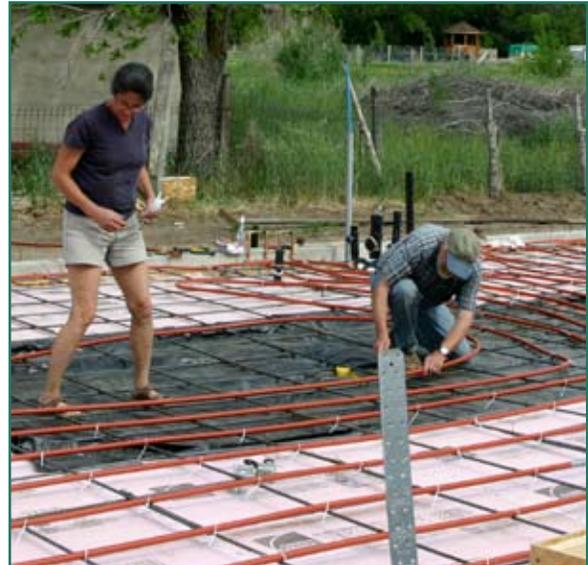
*Radiant heating system PEX tubing installed before pouring concrete slab. Zip ties are used to secure the tubing to the rebar. The ties are spaced close together to ensure that the tubing will not float to the surface when the concrete is poured.*
