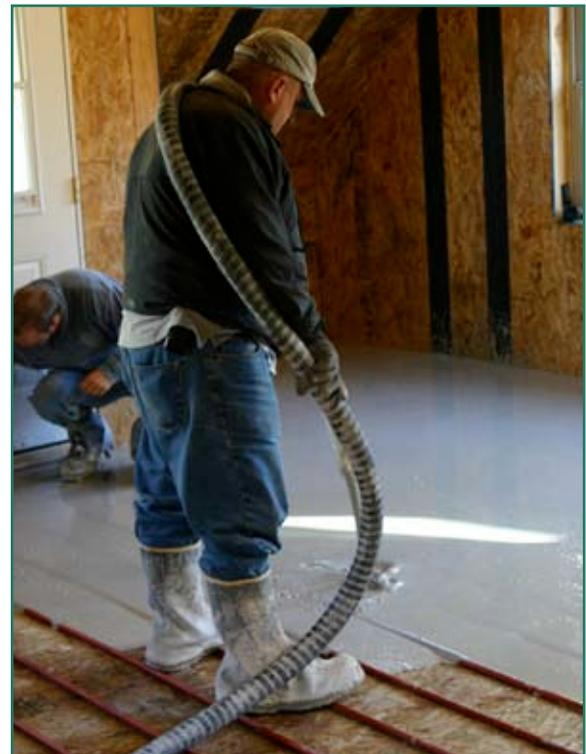
*Gypcrete poured onto second floor provides thermal mass for radiant heat tubing*
