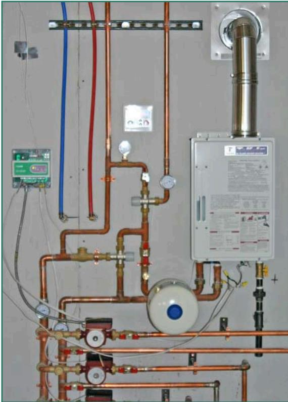
*Wall mounted tankless heater that provides domestic hot water and space heating for a 2,400 square foot building*
