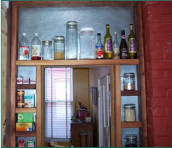
*Sheet metal used for open shelf backing*
