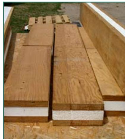
These insulated headers consist of foam cores sandwiched between LVL beams
