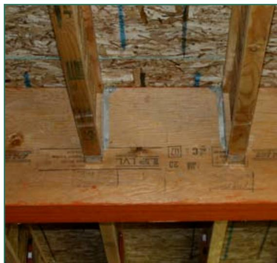
LVL beam with engineered floor joists
